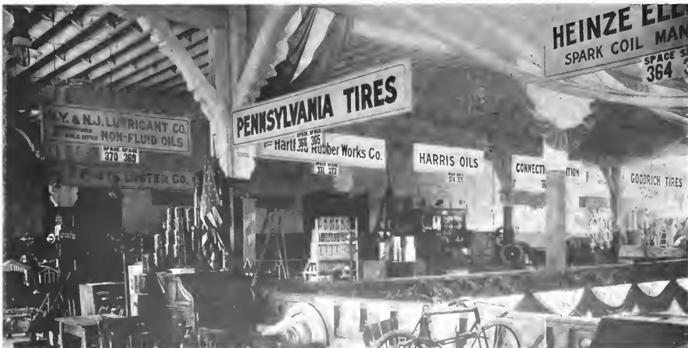
A Corner of the Second Floor, Where the Display of Accessories Was the Magnet That Attracted Many Visitors.
